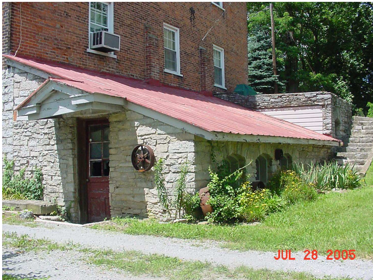
Photo of enclosed mill wheel building added to protect from weather. 2005. Photo taken by Jon Branstrator.
