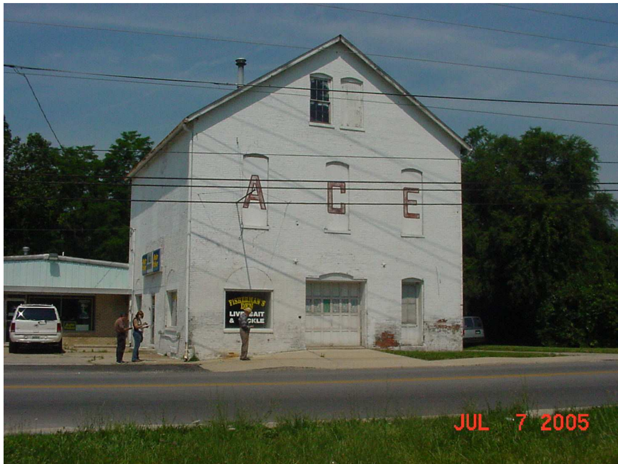
Moffitt Flour Mill. One of the two mills still standing in the county. 2005. Photo taken by Peggy Branstrator.
