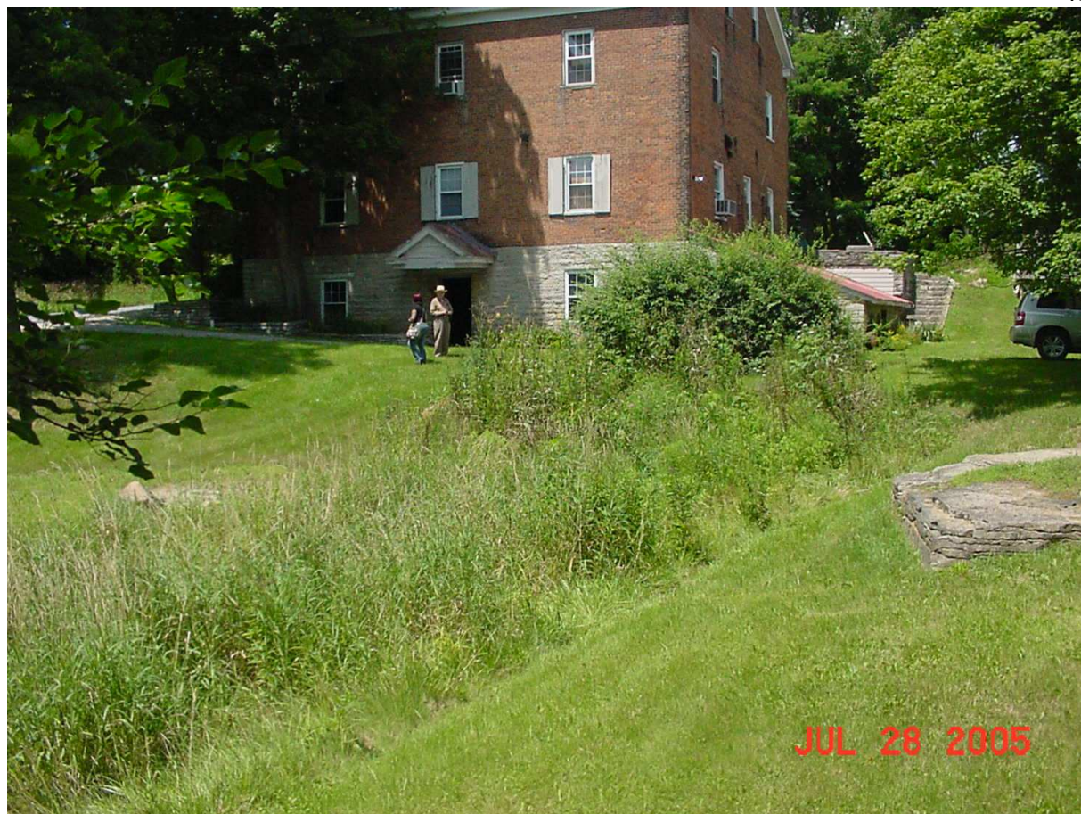
Photo of original raceway leading to mill. 2005. Photo taken by Peggy Branstrator.
