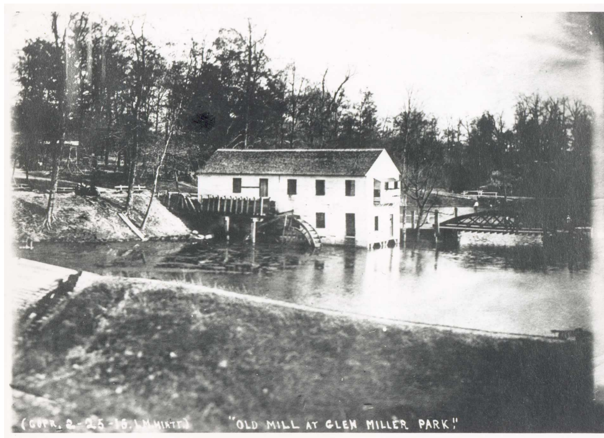
Hawkins Saw Mill after lake was formed. Picture taken before being torn down in 1880. Courtesy of the Indiana Historical Society.
